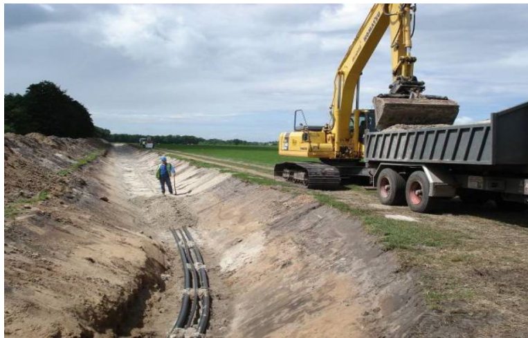
Figure 4. Example of Open Trench Construction
