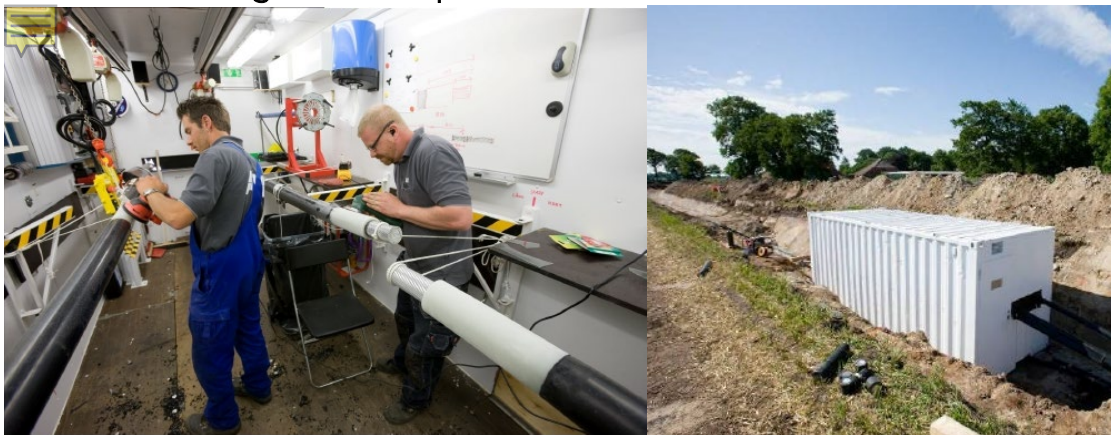
Figure 6. Example of HVDC Conductor Joint Construction
