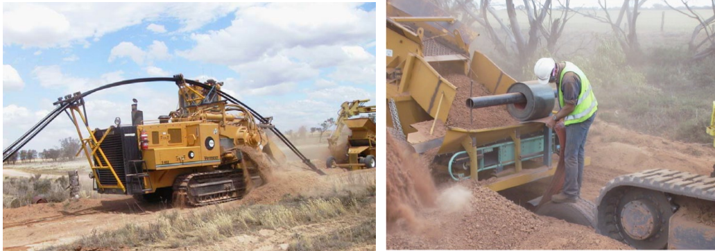
Figure 5. Example of Integrated Trench Construction
